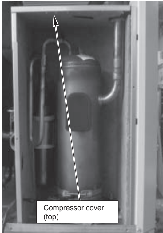
4. Remove the compressor cover (top).
